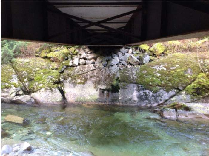
Right Bank Abutment when facing downstream
