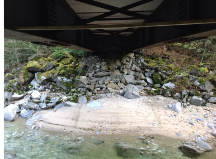
Left Bank Abutment when facing downstream
